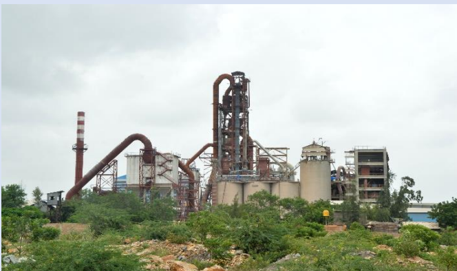
Capex 1 million Ton in Progress...
